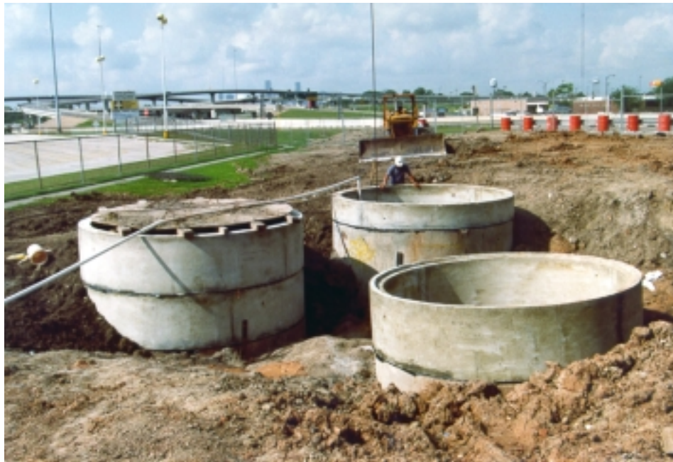
Figure 3-14. Circular caisson wet wells under construction.
