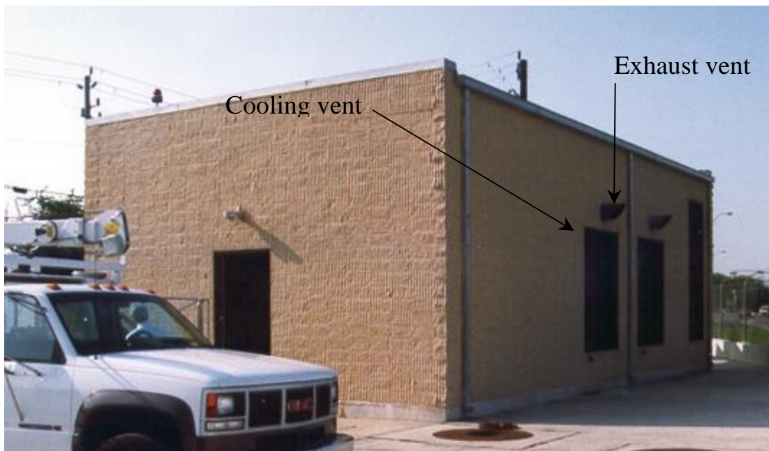
Figure 10-1. Typical pump house used by Texas DOT
