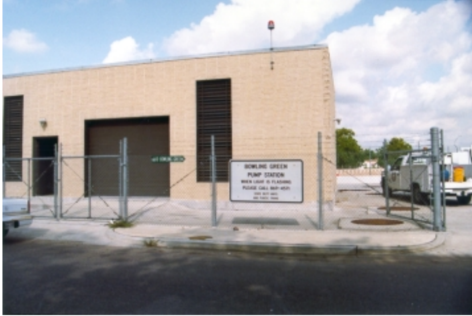
Figure 2-2. Highway stormwater pump house
