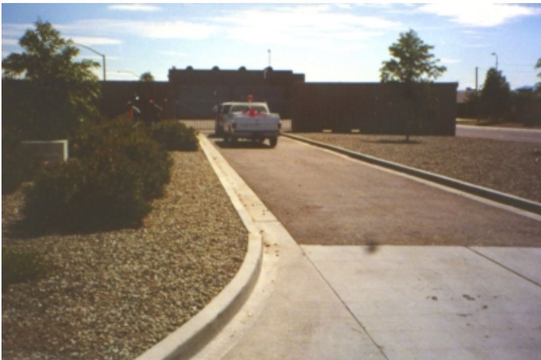
Figure 5-4. Driveway access to pump station in Arizona
