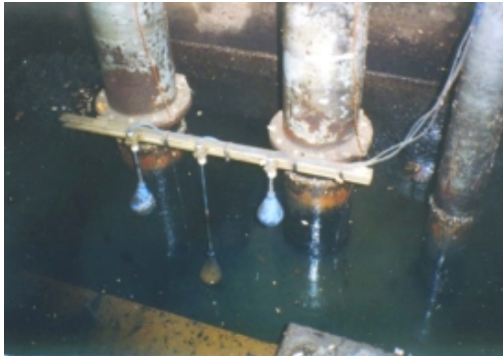
Figure 11-6. Tilting bulb switch
