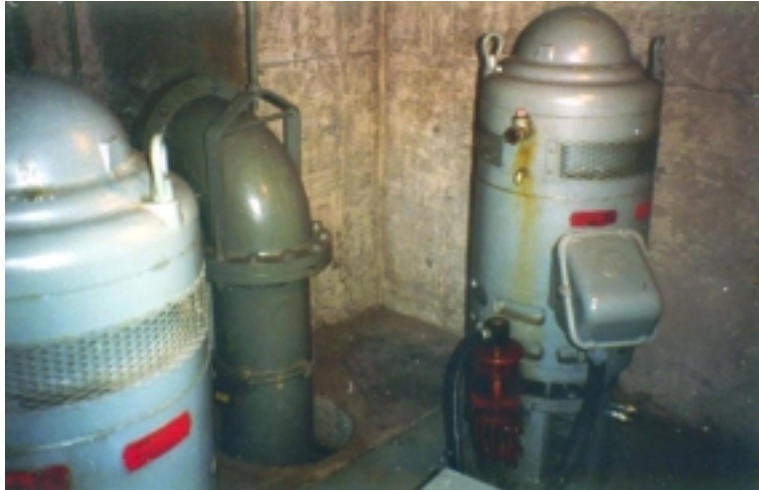
Figure 11-2. Typical electric motors for vertical pumps
