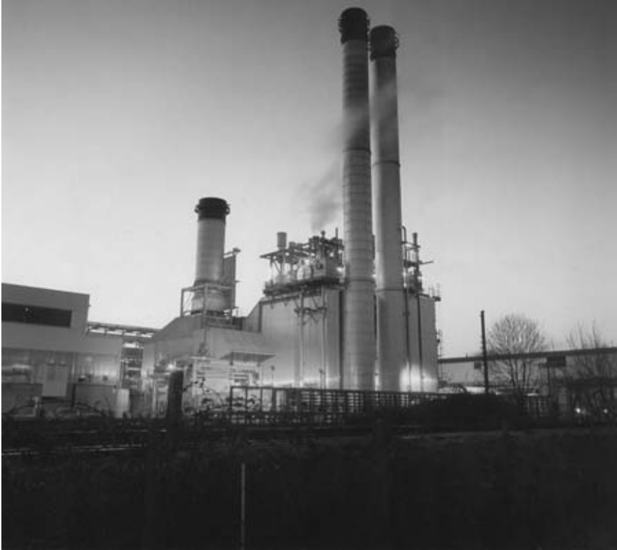
Aylesford Co-generation Plant The plant produces 220 MW heat and 98 MW of electrical energy [National Power PLC]
