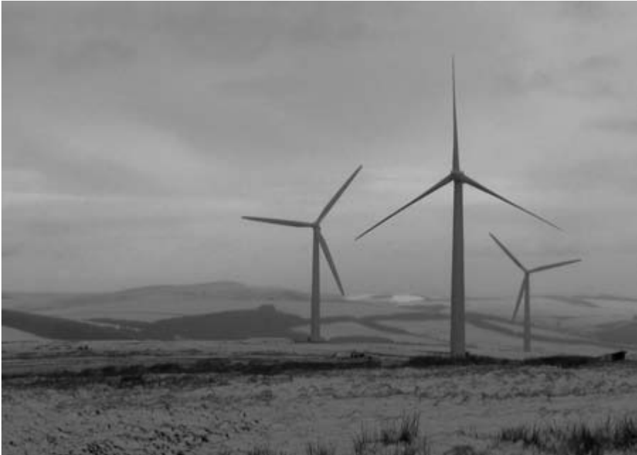
Black Hill Wind Farm, Duns, Scotland (28.6 MW) [RES]
