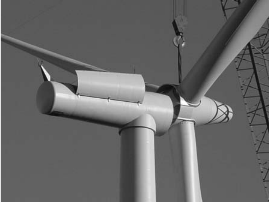
Nine Canyon Wind Farm, Tri-Cities, Washington USA (100 MW) Attaching the blade assembly of a 1.3 MW, active stall regulated, fixed speed induction generator wind turbine [RES]
