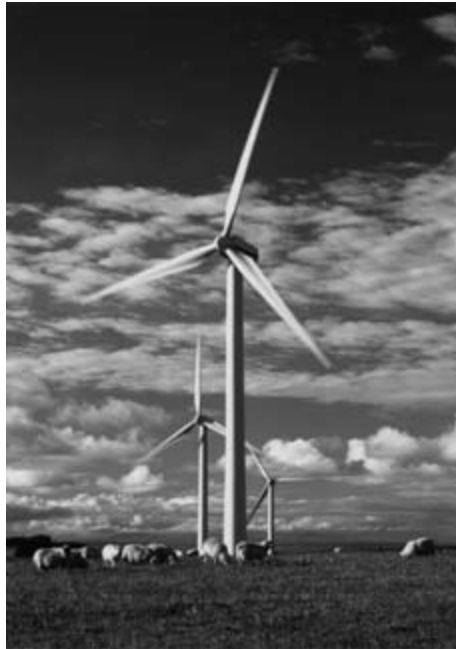
Dun Law Wind Farm, Oxtou, Scotland (47 MW) Turbines are pitch regulated, variable speed using Doubly Fed Induction Generators [RES]
