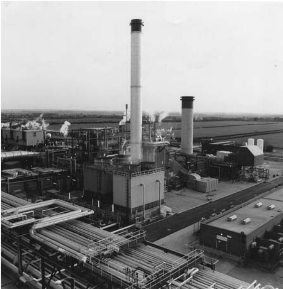
Lindsey Oil Refinery Co-generation Plant The plant produces 118 MW heat and 38 MW of electrical energy [National Power PLC]
