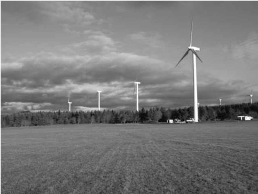
Plateau Ardéchois Wind Farm, Rhône Alpes, France (6.8 MW) 850 kW Doubly fed induction generator wind turbines [RES]
